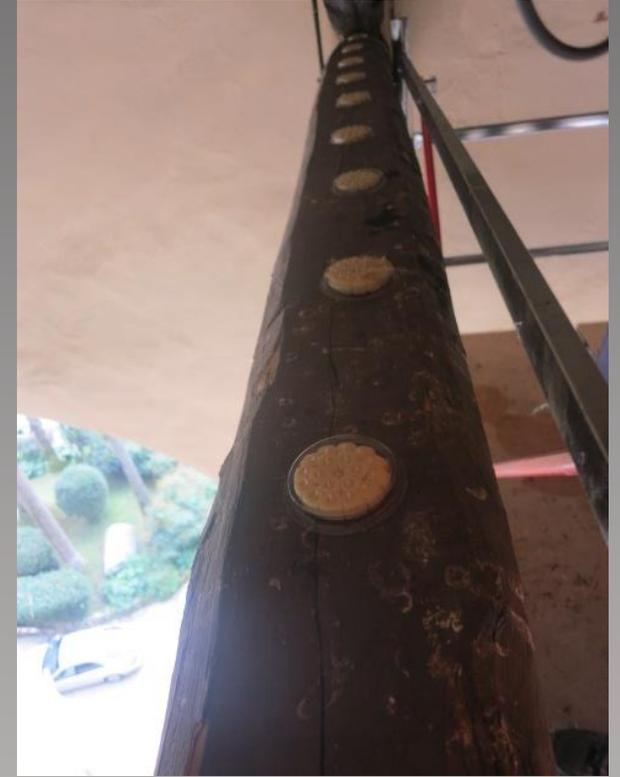
The seven delta-shaped rafters in the south section of the loggia were first cleaned. Dishes of 小島 *Bird Free* were then fitted to the upper parts of the rafters at 20cm centres (above middle), and to the lower part of the rafters at 25cm centres (above right). The dishes are invisible from below.
