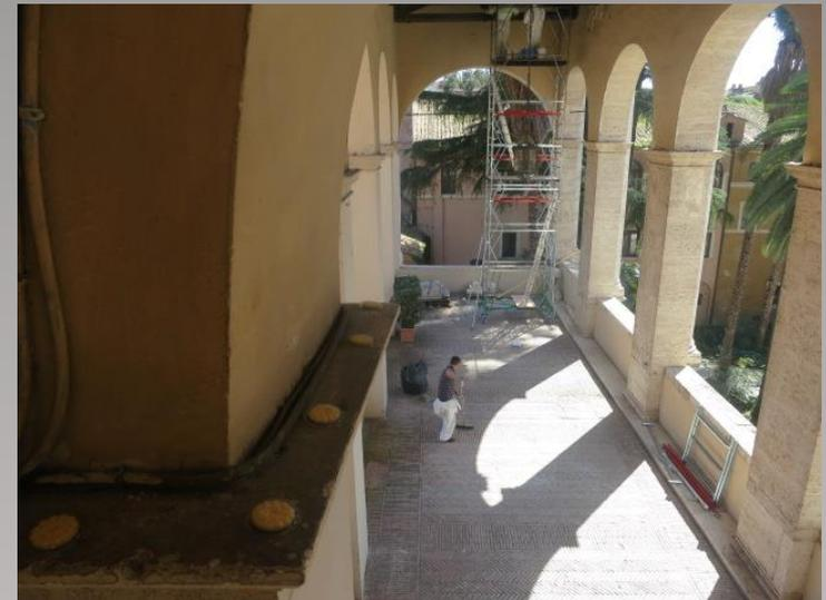
Dishes of 小島 *Bird Free* were fitted at 25cm centres to all small ledges on both sides of the L-shaped loggia to prevent displacement.
