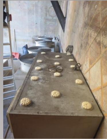
The ledges and air conditioning equipment inside the inner courtyard were treated with dishes of 小島 *Bird Free* as shown above.
